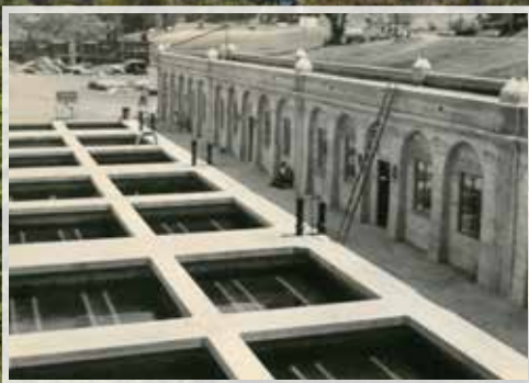
Orinda Water Treatment Plant under construction
