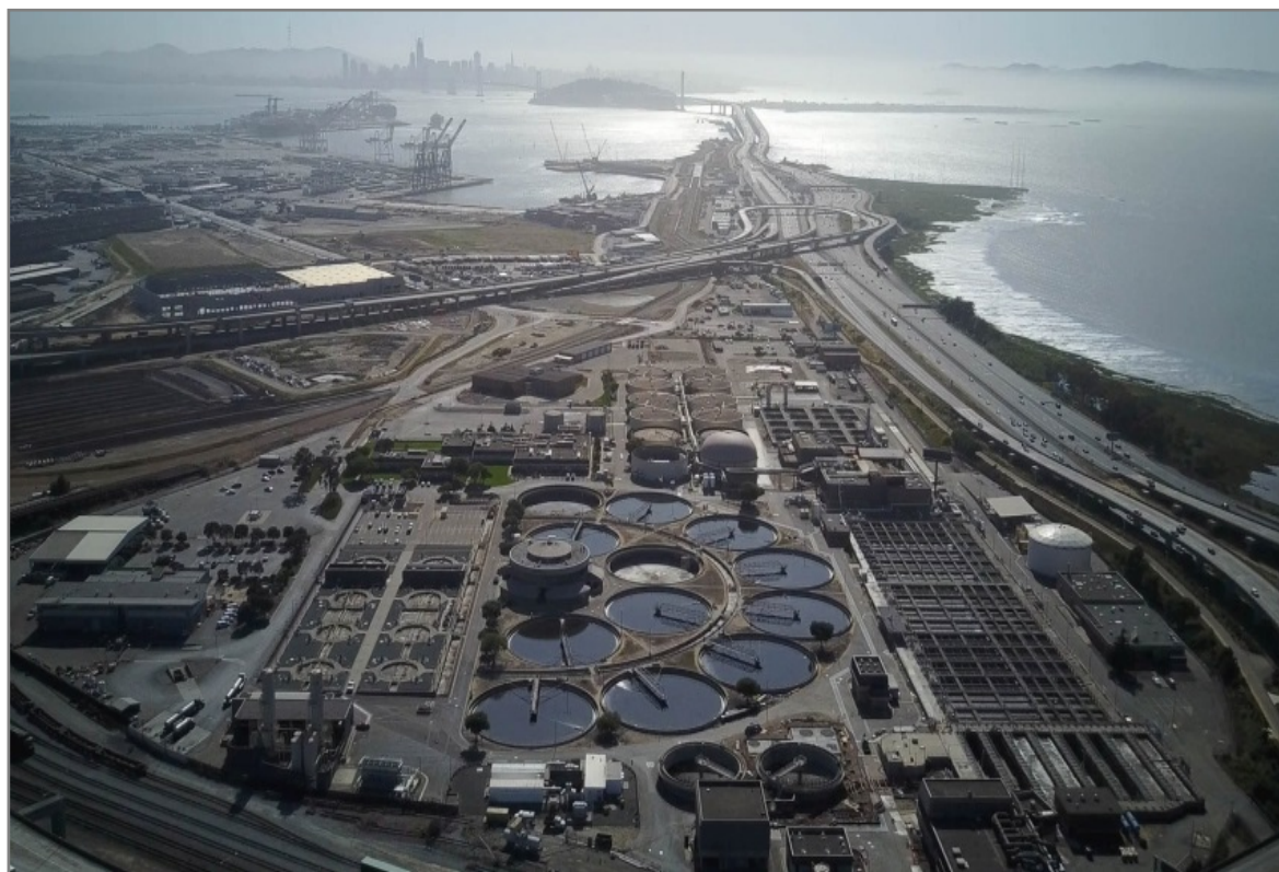
Wastewater Treatment Plant – Oakland, CA
