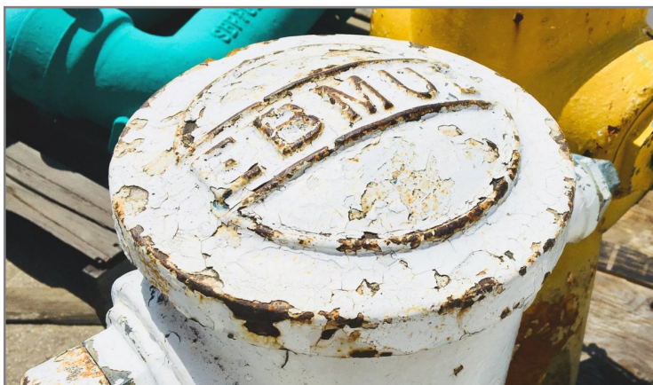
Old 1890-Style Fire Hydrant
