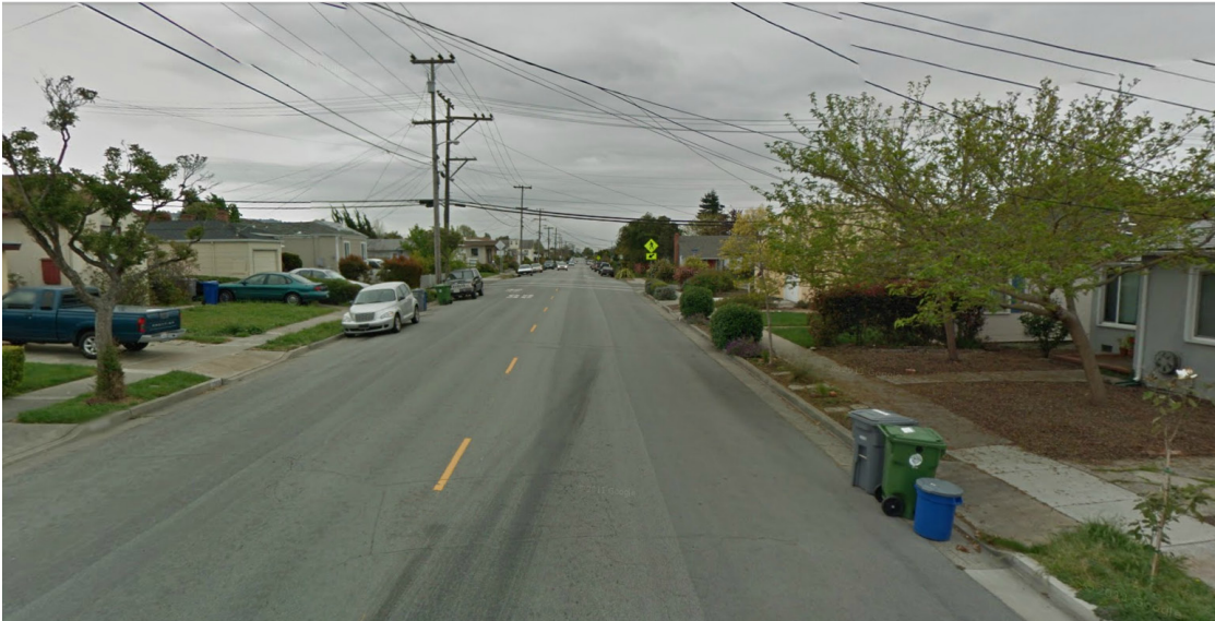
Photo 3: Typical residential area along Richmond Street.
