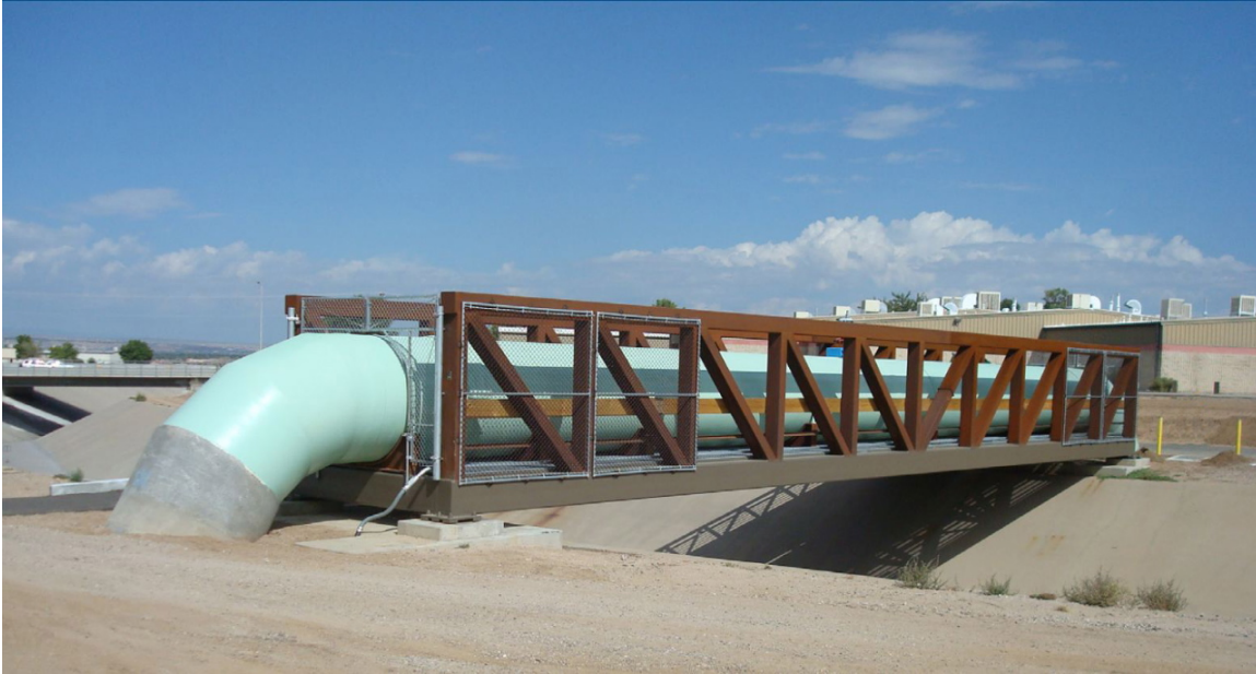
Figure 2-14 Typical Pipe Bridge Construction
