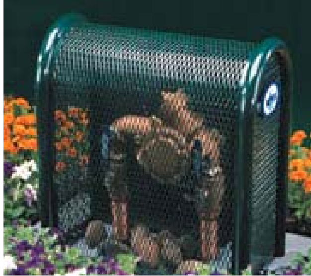
Figure 2-10 Typical Air Valve
