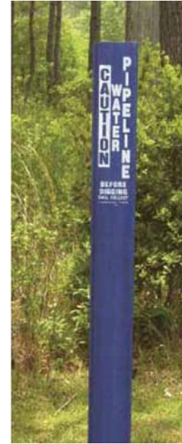
Figure 2-11 Typical Marker Post
