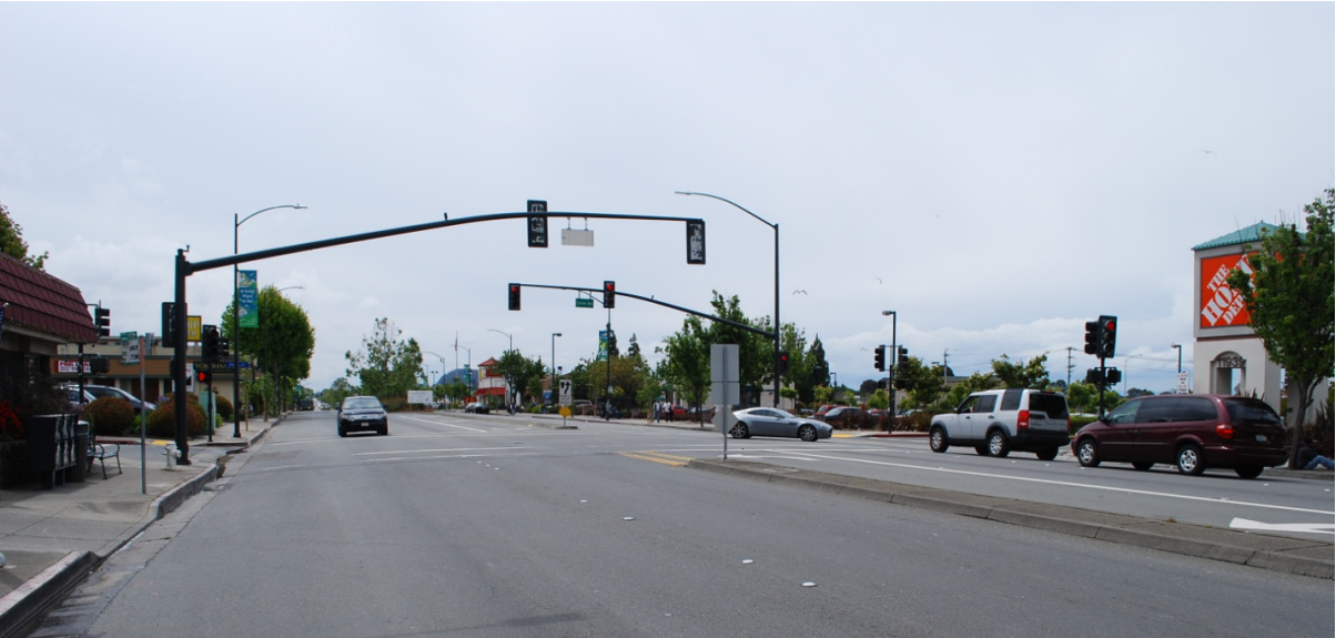
Photo 7: View of San Pablo Avenue near the northern end of the proposed alignment.
