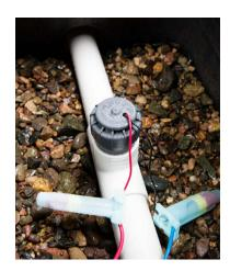
2) Wiring to correct sensor port in controller and image showing connected/active flow sensor.
