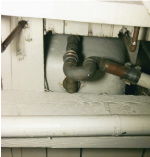
The shower p-trap is the copper pipe shaped like the letter “p.” In this example, the p-trap and shower drainage pipes are visible below the shower/tub. Photo: Josh Lowe.
