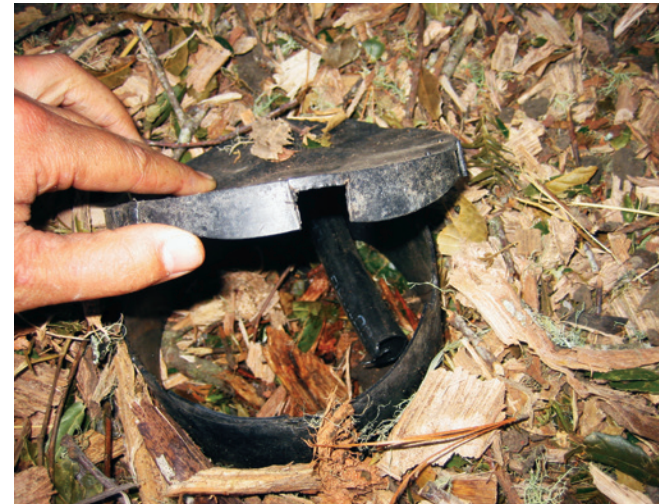
Cut a 6-inch section from the drain pipe and drill a hole 2 inches below the top for the graywater tube to enter. Cover the open top with a paver or tile.
