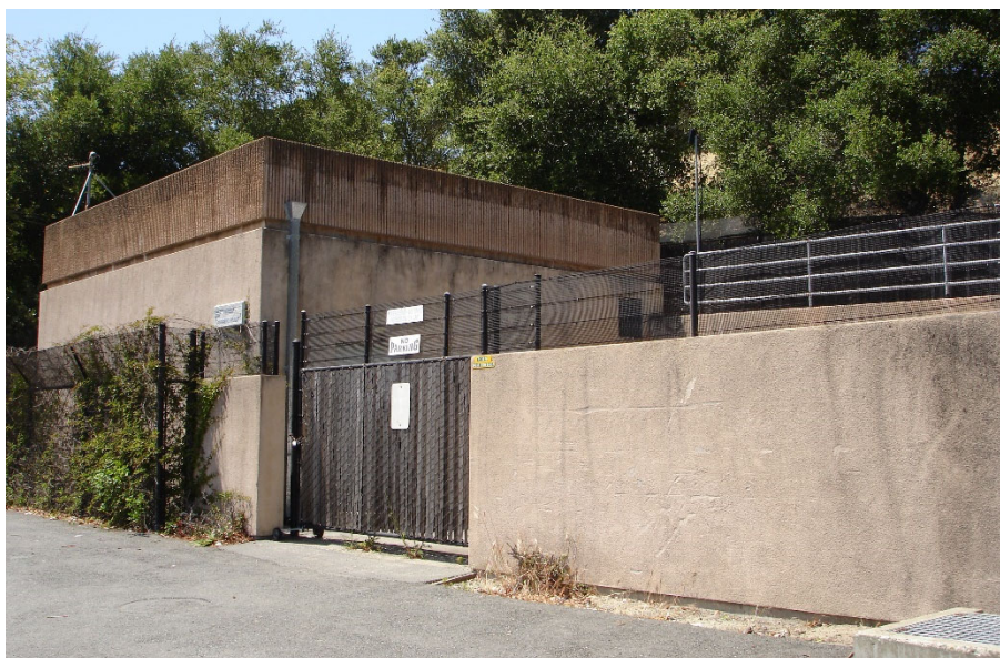
Example Installation of CMU Wall
