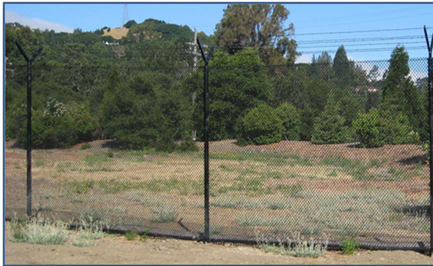
Example Installation of Security Chain Link Fence
