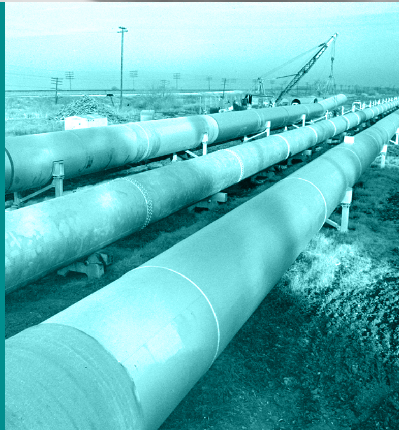
Mokelumne Aqueduct #3 under construction, 1963
