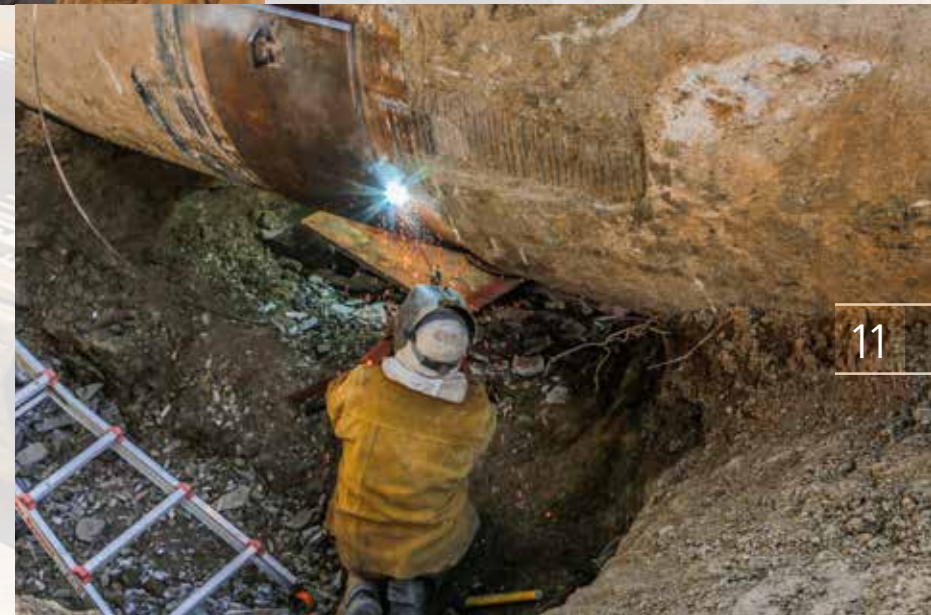
EBMUD welder Artur Amaral at work repairing an aqueduct in Walnut Creek.
