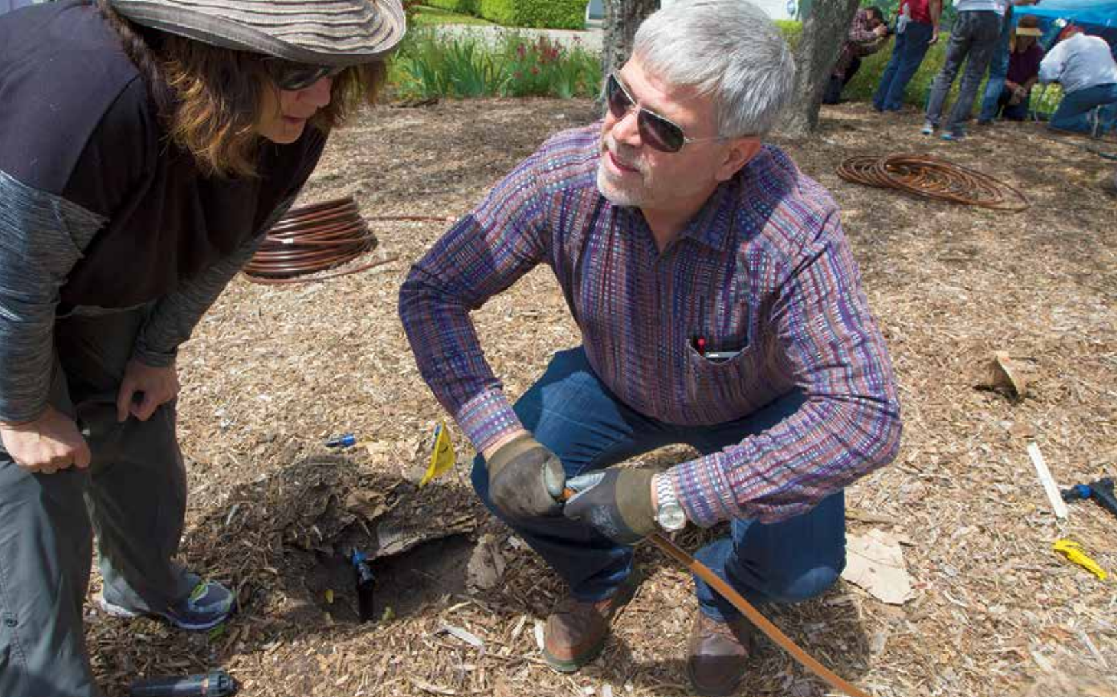
Conservation expert Scott Sommerfeld shows gardeners how to install in-line drip irrigation, a more efficient option to water landscapes.
