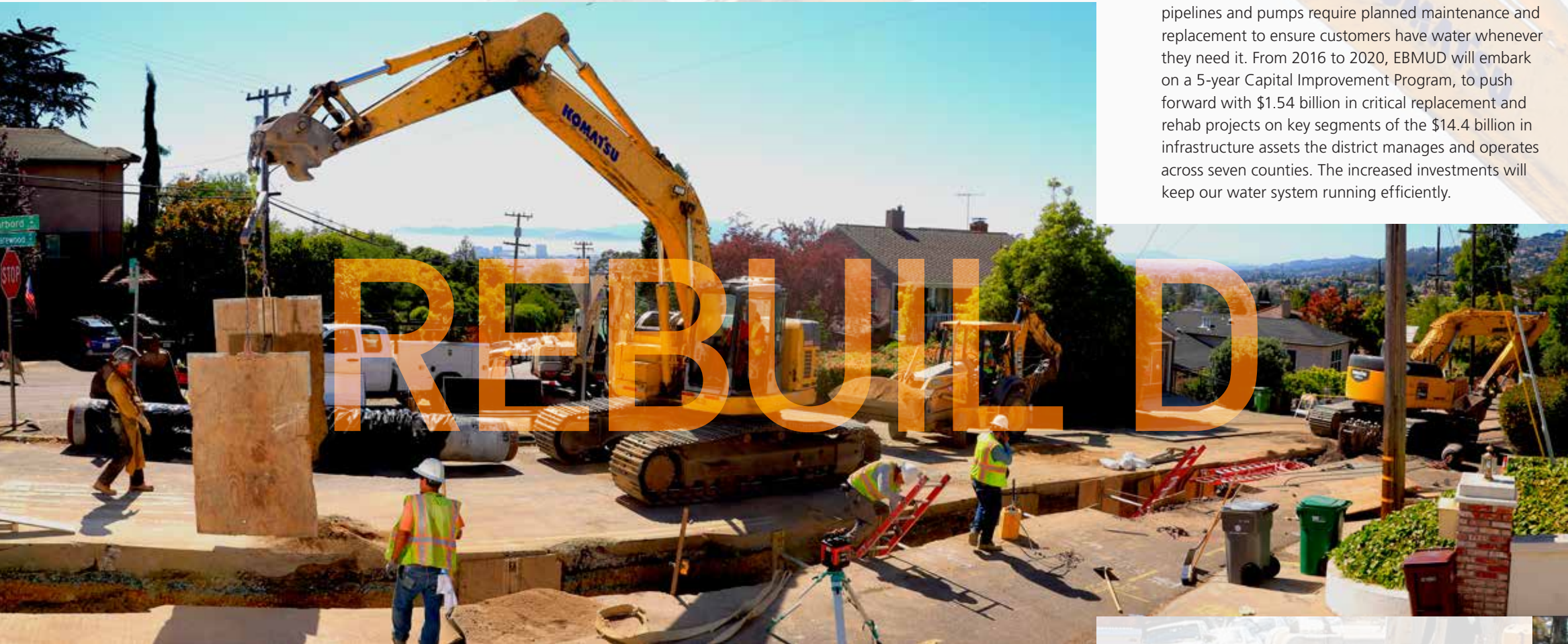
EBMUD replaced an aging 12,000-foot segment of pipe that delivers water to customers in the central Oakland Hills.
