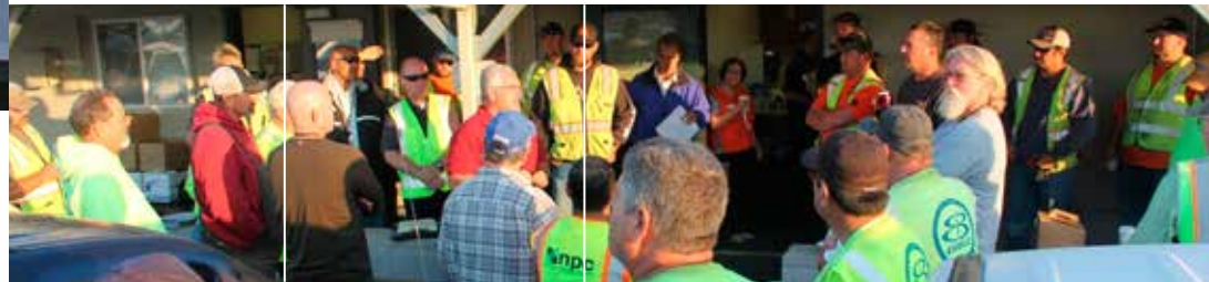
EBMUD crews repaired main breaks in the City of Napa following the magnitude-6.0 earthquake; the Bay Area's strongest in 25 years.
