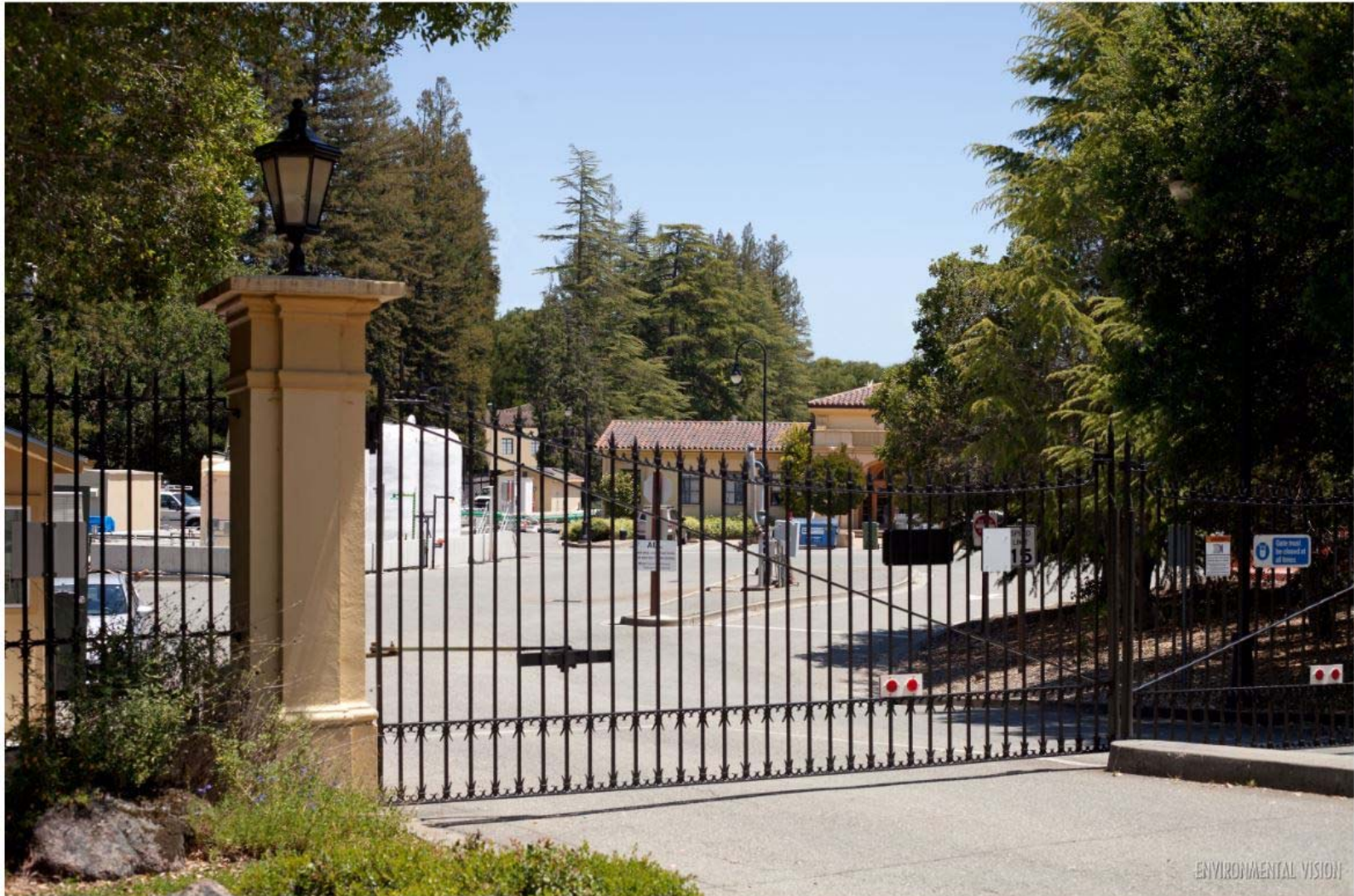
Visual Simulation with Project View from Manzanita Drive at Orinda WTP north entrance
