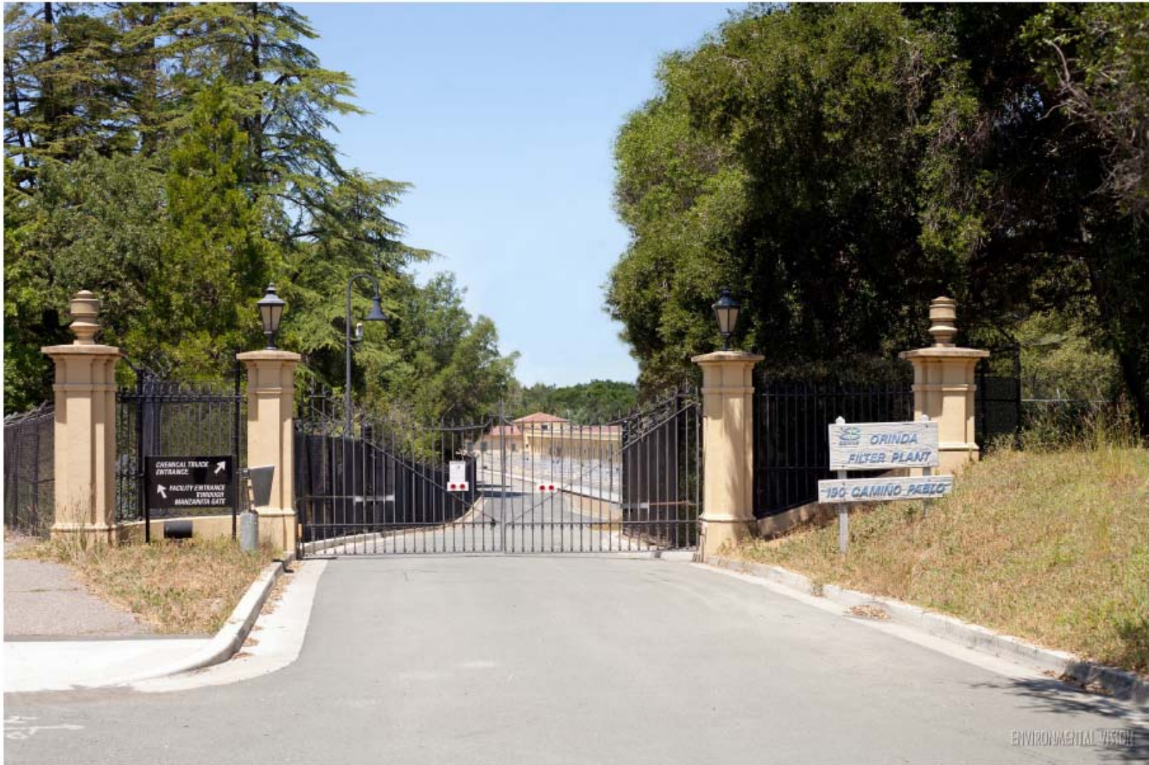
Visual Simulation with Project | 5-Year Projection View from Camino Pablo at Orinda WTP south entrance
