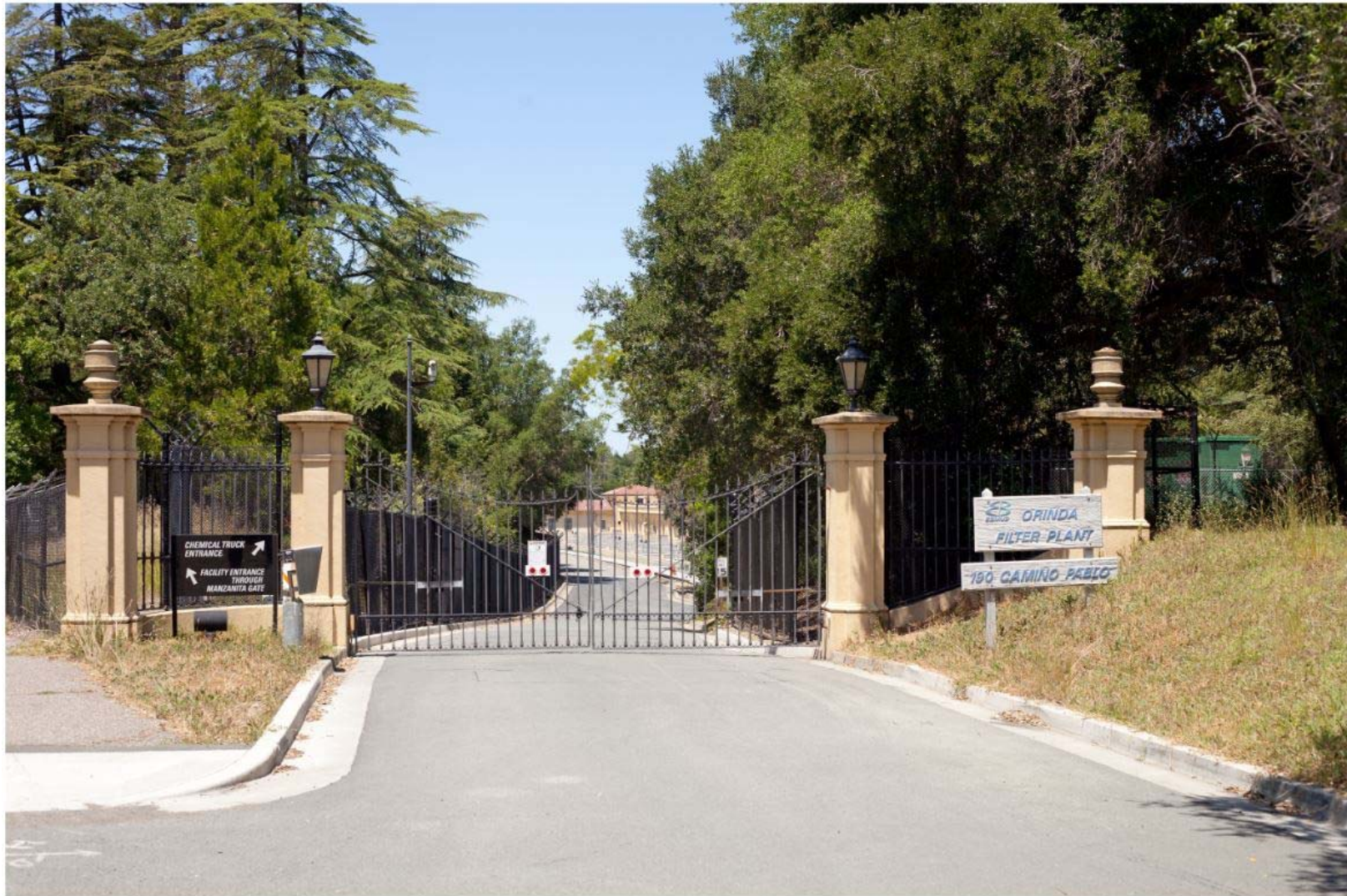
Existing View from Camino Pablo at Orinda WTP south entrance (VP 1)
