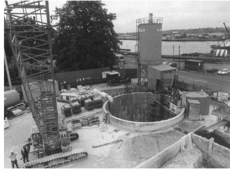
TYPICAL TUNNEL ENTRY SHAFT CONSTRUCTION SITE
