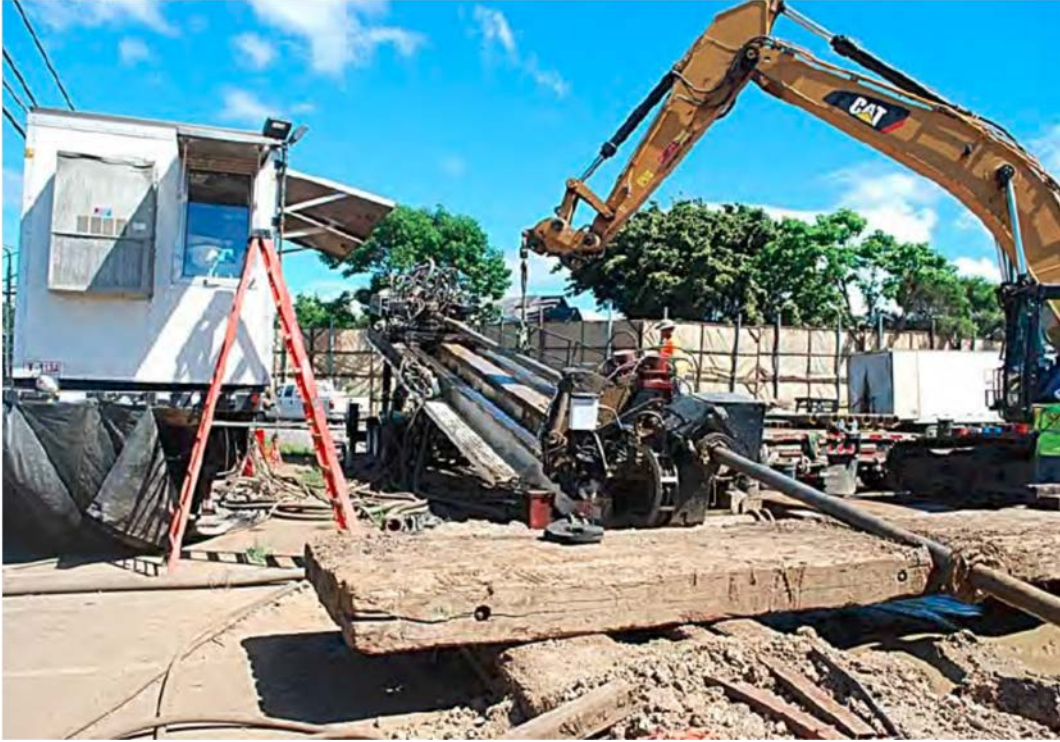
Equipment Associated with HDD
