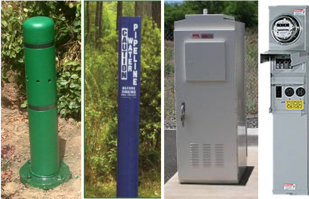
Figure 2.6-1 Above Ground Appurtenances: Air Valve Vent, Marker Post, RTU Cabinet, and Electrical Service Panel
