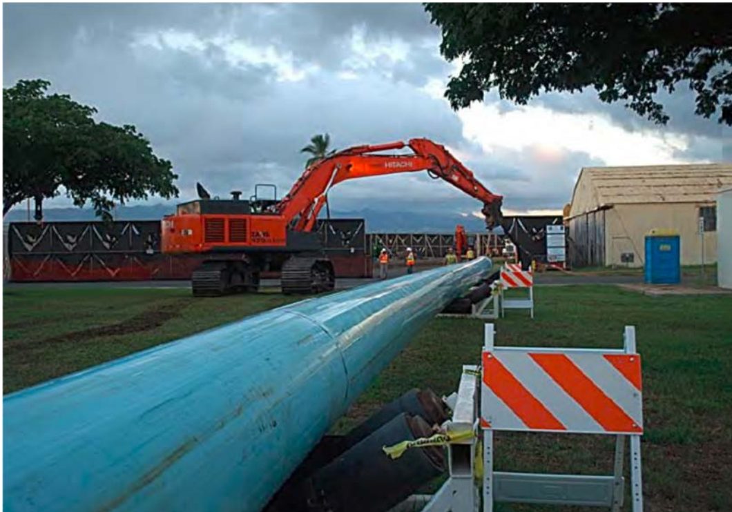
Pipeline and pulling equipment
