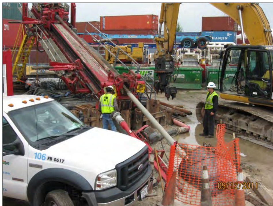
Figure 4-5. HDD Setup with Surface Conductor Casing
