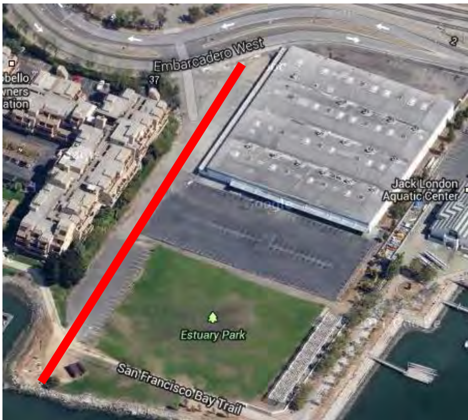
Figure 9: Fallon Road Terminus at Crossing 1D
