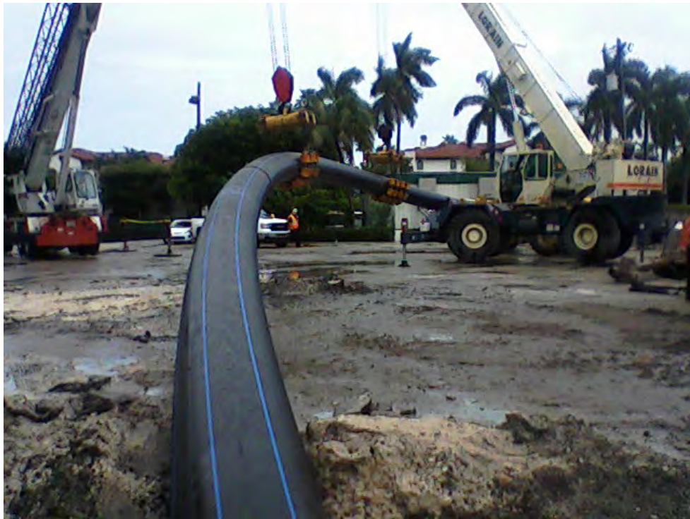
Figure 4-8. 24-inch ID HDPE Pipe Being Pulled into the Final Hole
