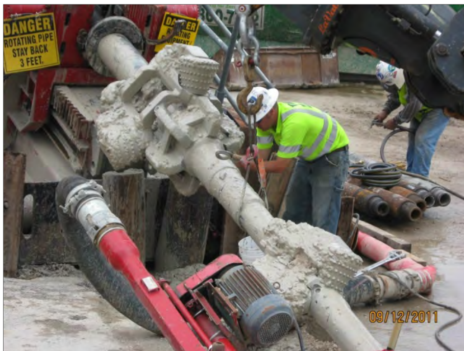
Figure 4-7. HDD Reaming Tools
