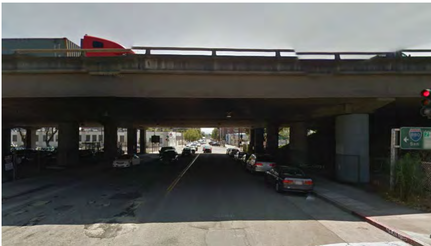
Figure 15: Highway 880 (Nimitz Freeway) Crossing at Jackson Street
