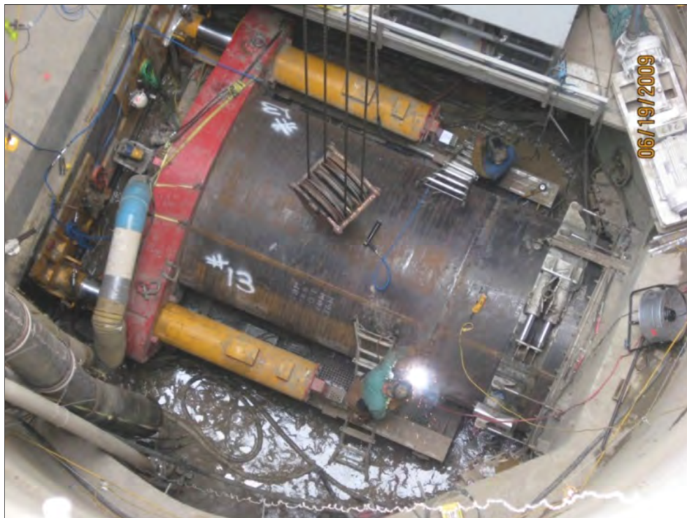
Figure 4-2. Placing Pipe for Jacking during Microtunneling Operation
