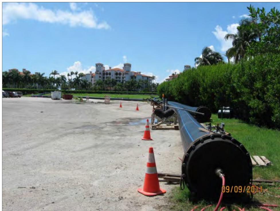
Figure 4-9. Pre-installation Pressure Test on Fused HDPE Pipe
