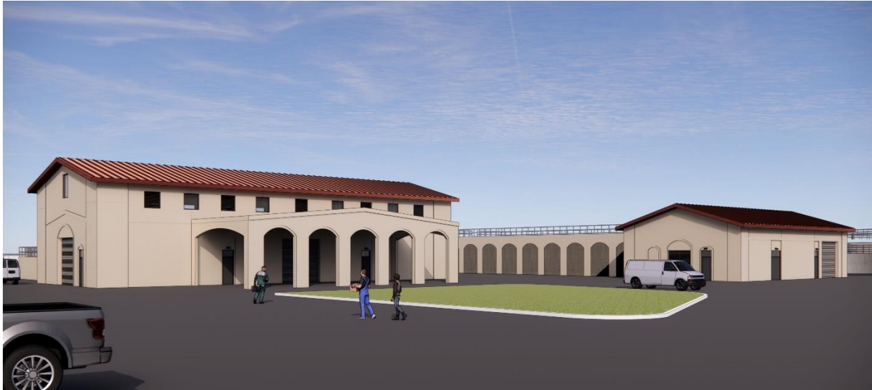
Figure 5.5.3: View of Buildings in Area A
