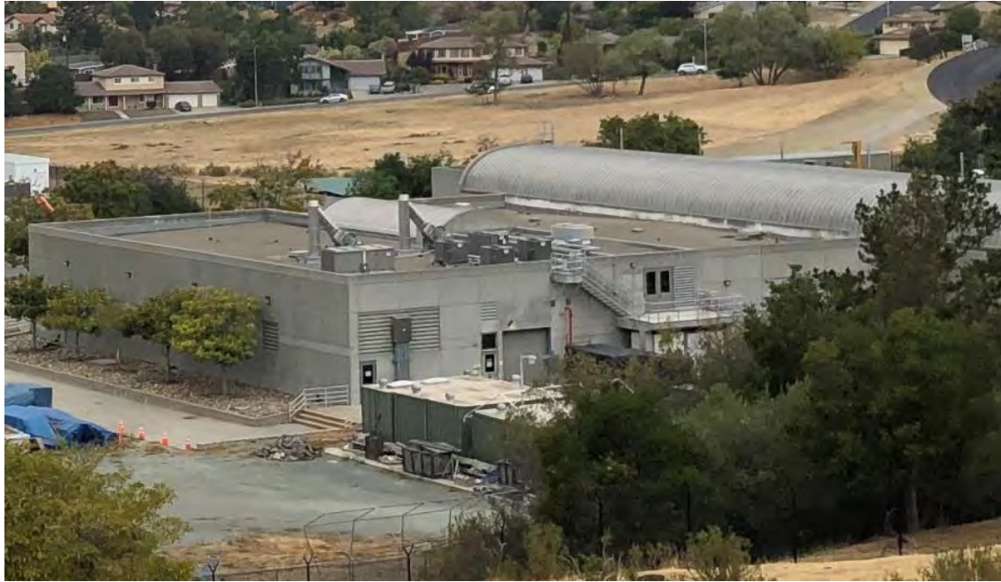
CHEMICAL & OZONE BUILDING
