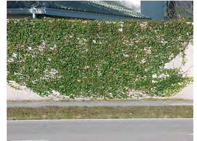
Concrete wall with vine planting
