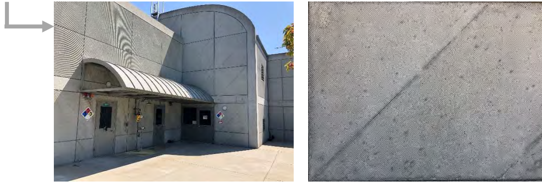
CHEMICAL & OZONE BUILDING CONCRETE PATTERN
