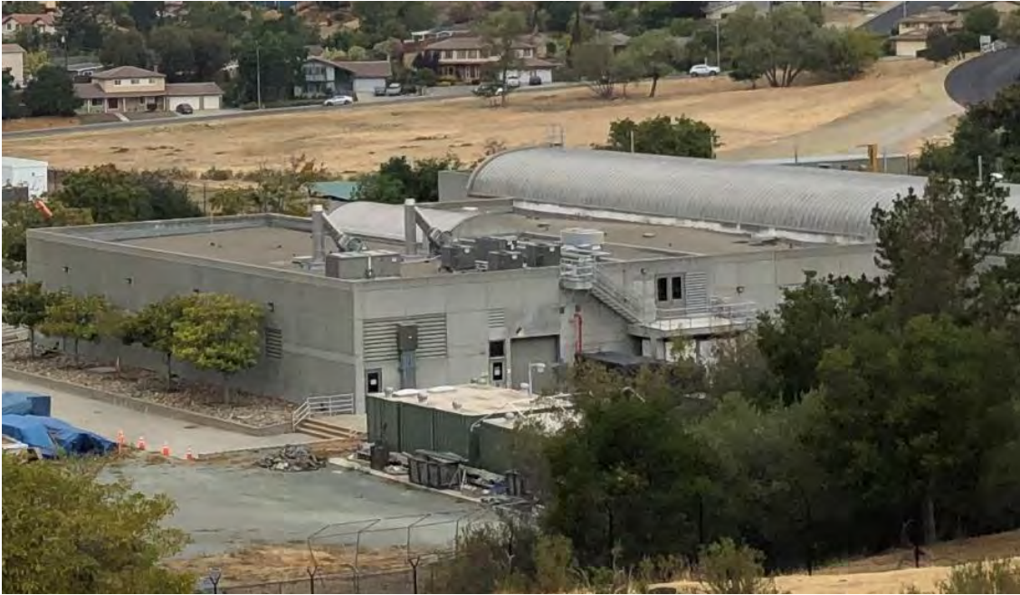
CHEMICAL & OZONE BUILDING
