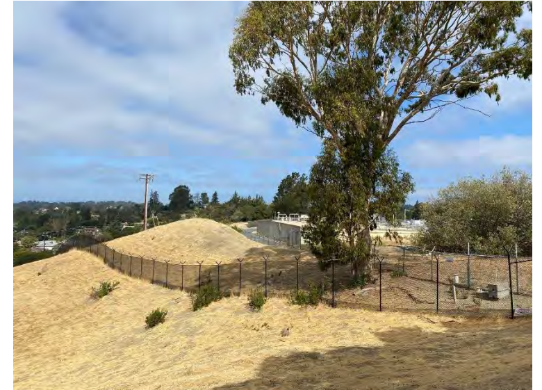
Spanish Trails – Side view showing berm construction
