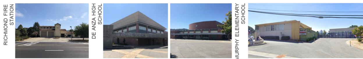
Figure 2.2.1 Visual Survey of Key Area Public Buildings
