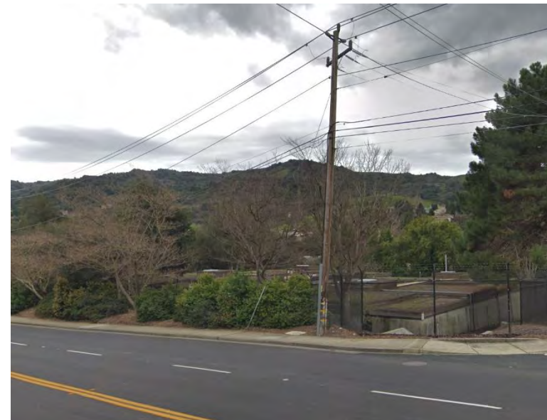
Valley View Road & De Avila Way – Low shrubs screen equipment
