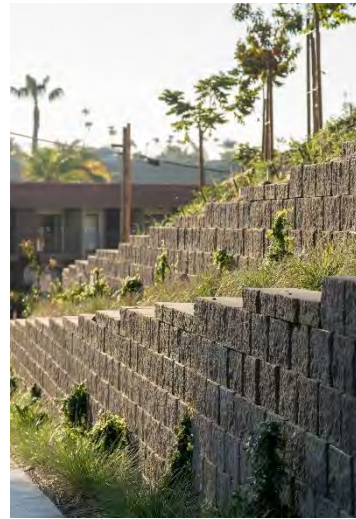
Berm and wall combination
