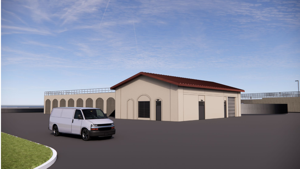
Figure 2-7 Power and Polymer Building
