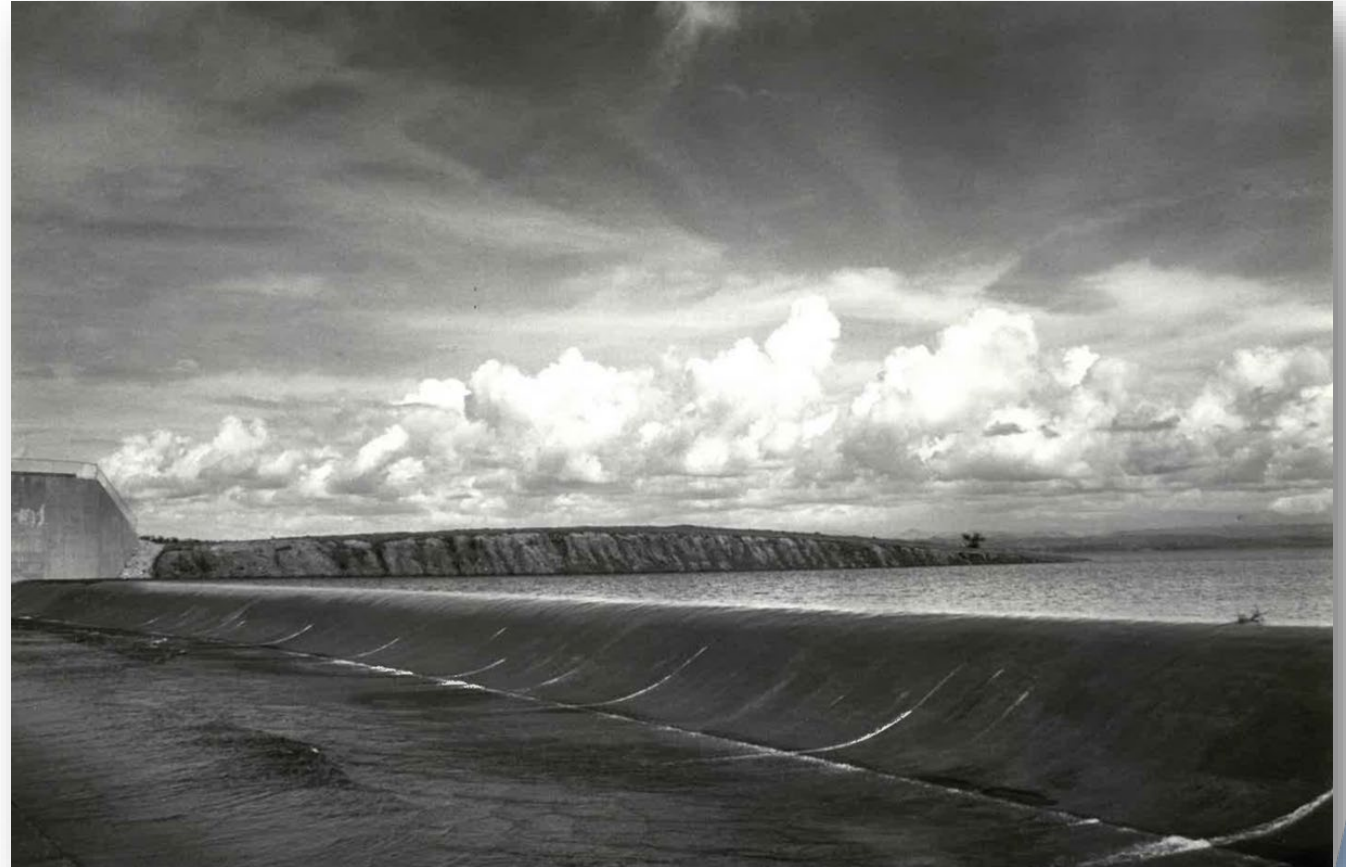
Camanche Spillway, February 1986 Peak Spill 1,630 cfs
