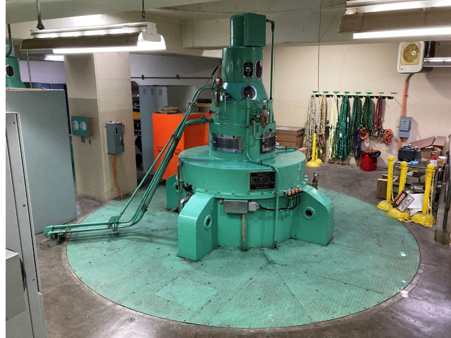
Current Condition (Unit No. 3)
