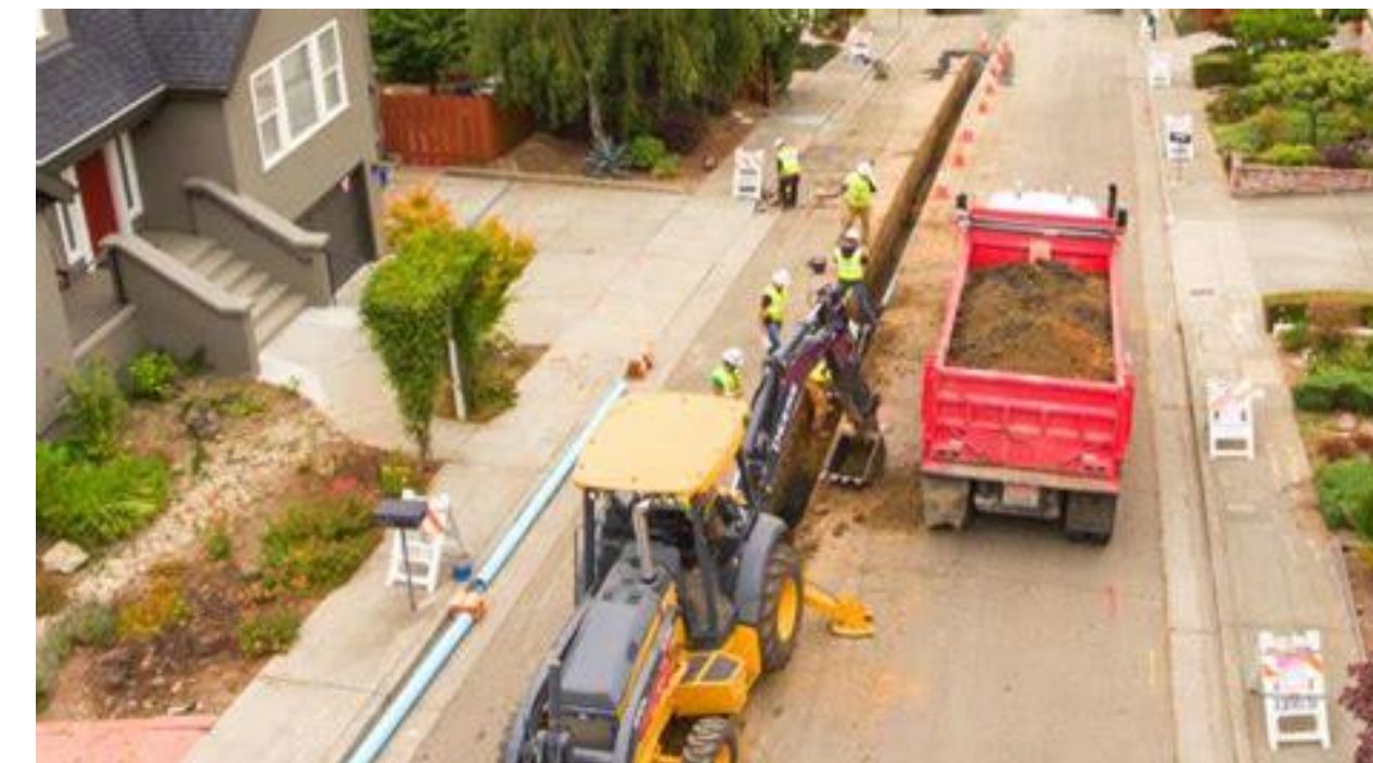
Open Trench Construction
