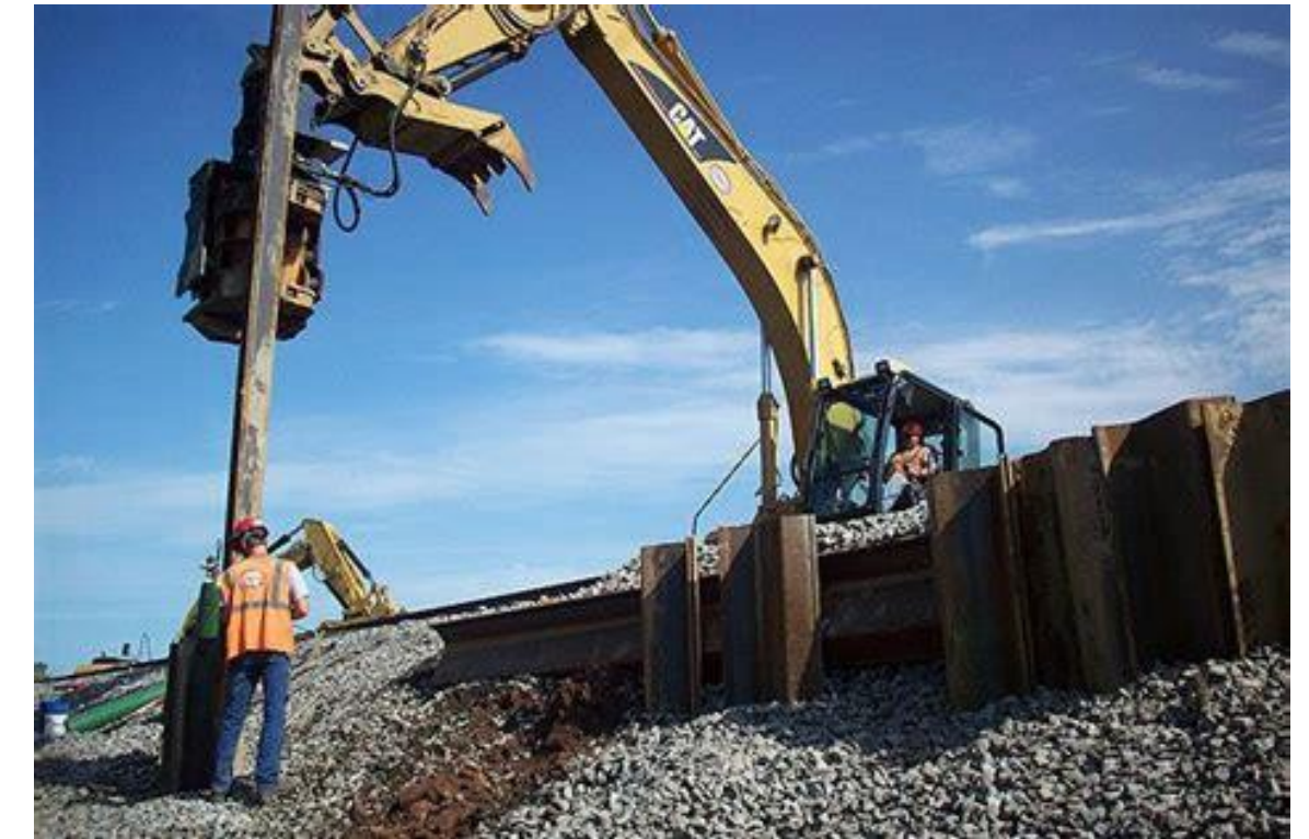
I-Beam Installation
