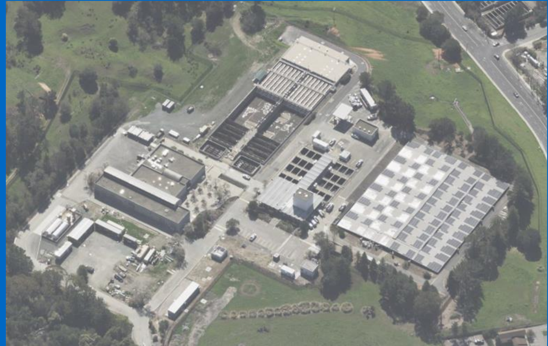
Sobrante Water Treatment Plant
