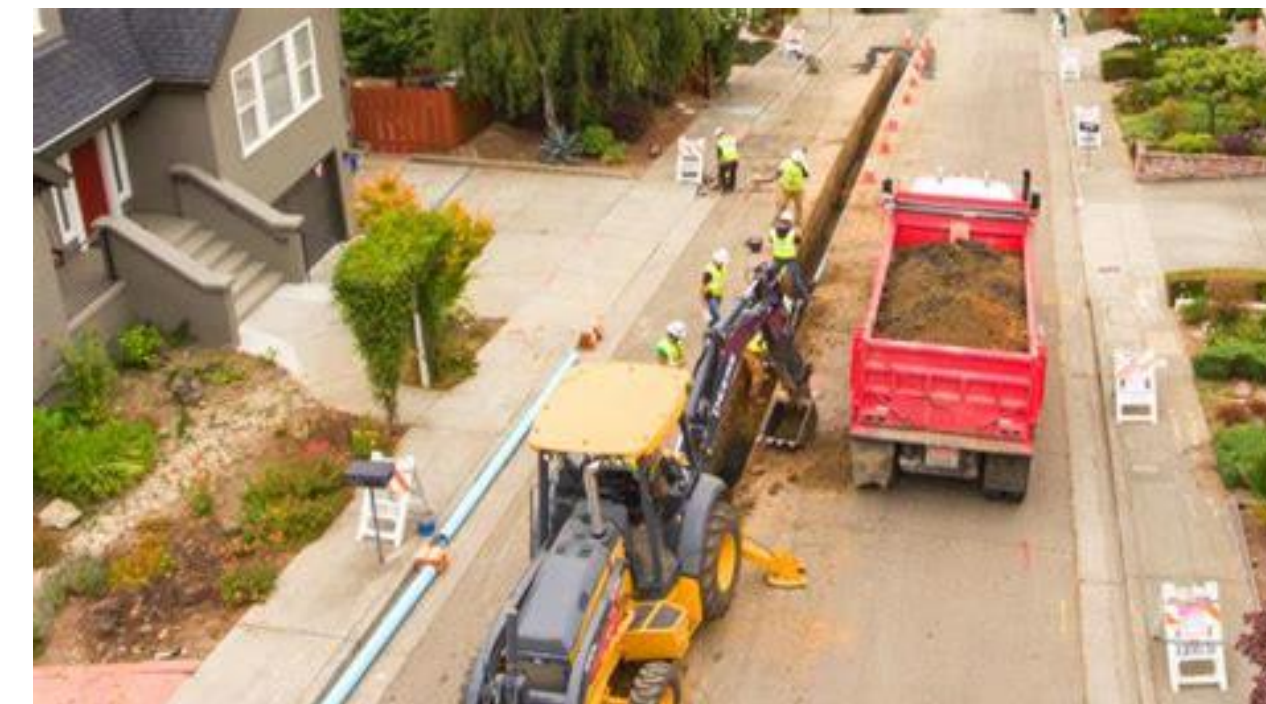
Open Trench Construction
