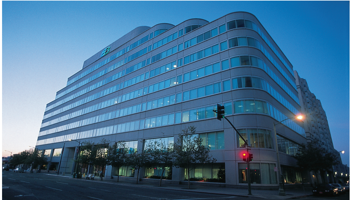
EBMUD Administration Building in downtown Oakland.
