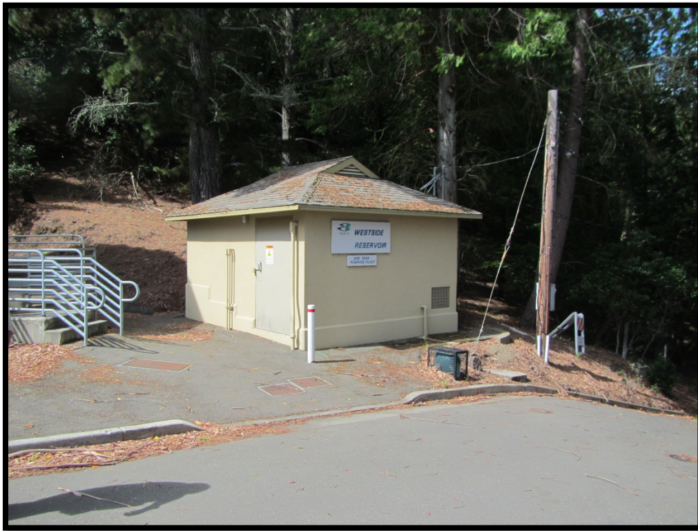
Photo 6. Dos Osos Pumping plant located at Westside Reservoir, facing west
