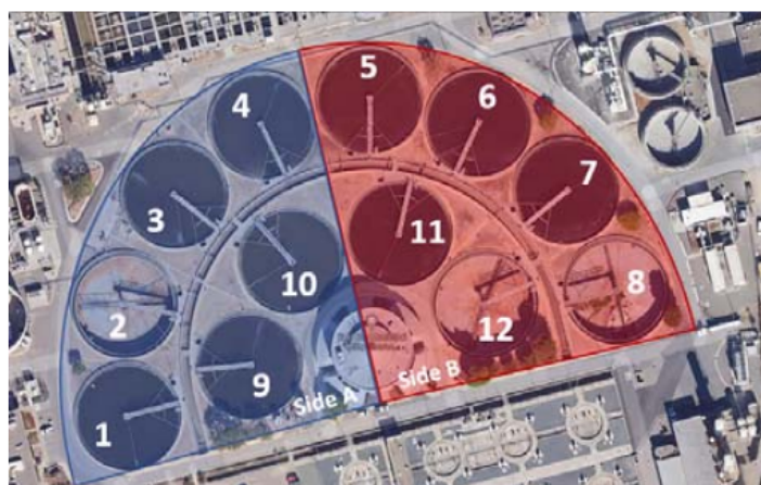
Figure 1-1: MWWTP Secondary Clarifiers
