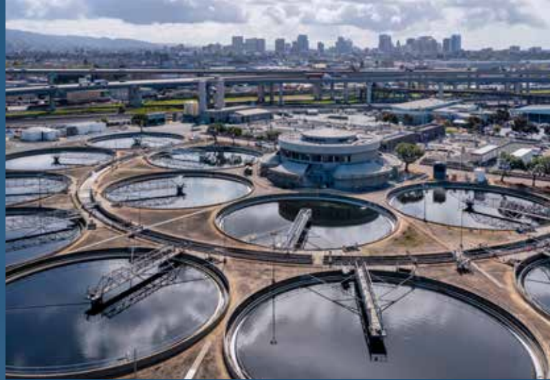
Our wastewater treatment plant operates around the clock every day of the year.
