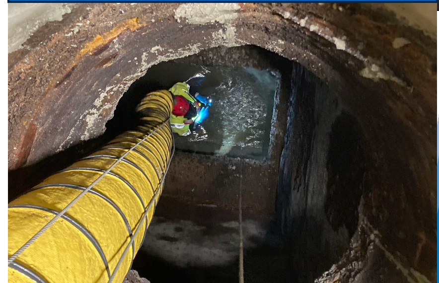
Corroded Maintenance Hole
