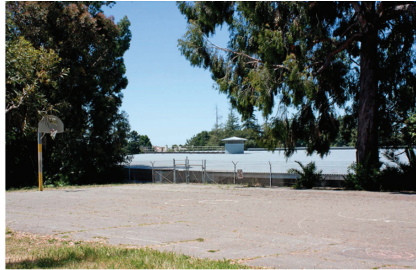
Photo 8: Central Reservoir Recreation Area at basketball court looking southwest, towards east portion of site
