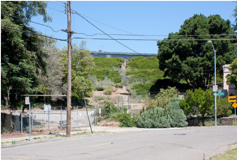
Existing View - 25th Avenue near East 29th Street looking north (Photo 3)
