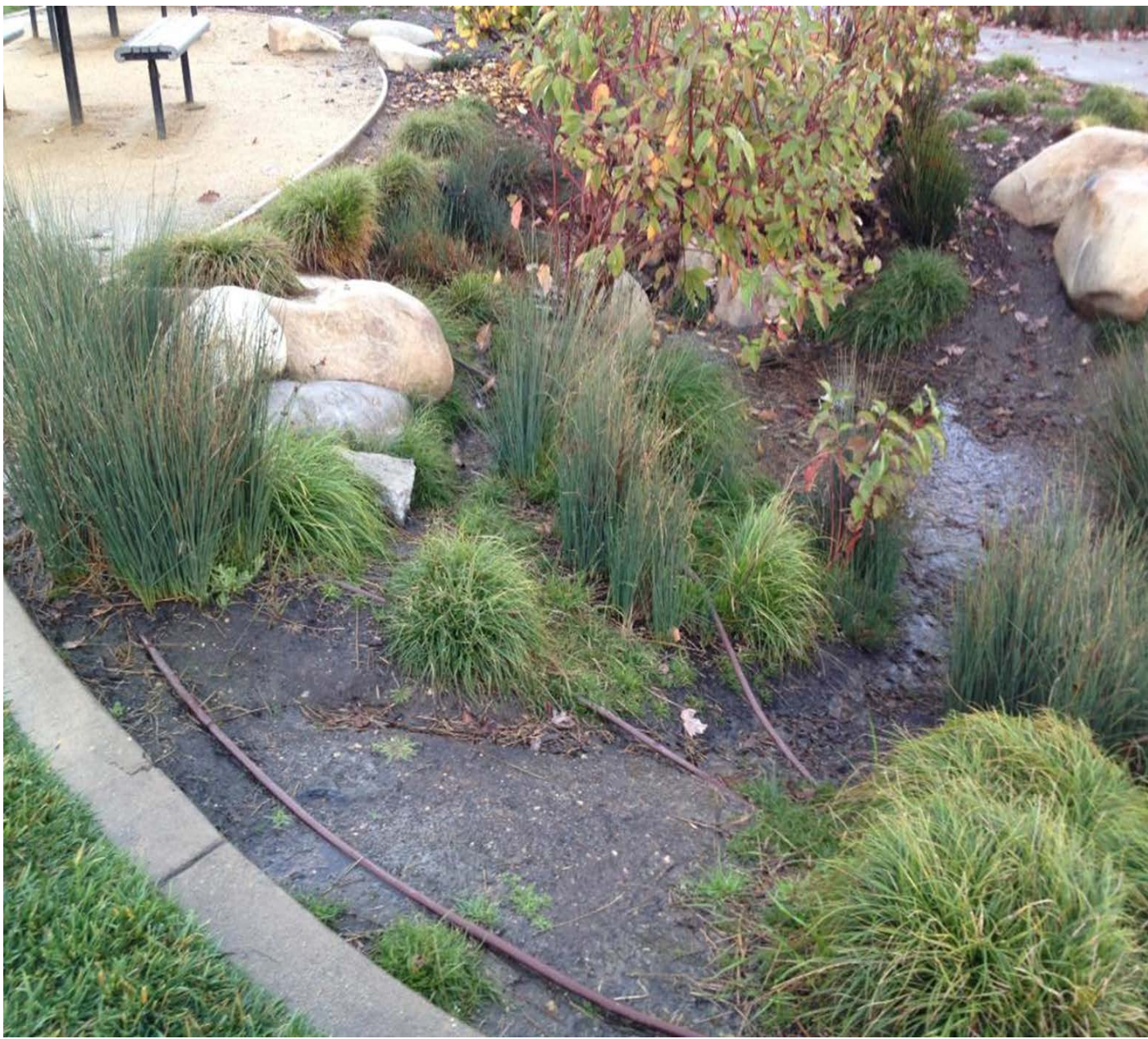
A Bioretention Area...
