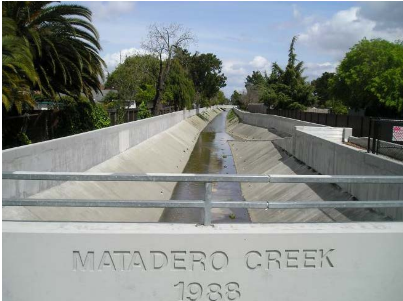
Concrete Lined Channel with Floodwall in Lower Matadero Creek
