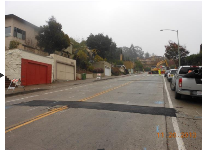
Paving Over Trench
