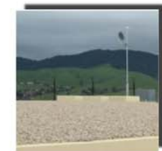
Gravel Rock Roof Treatment
