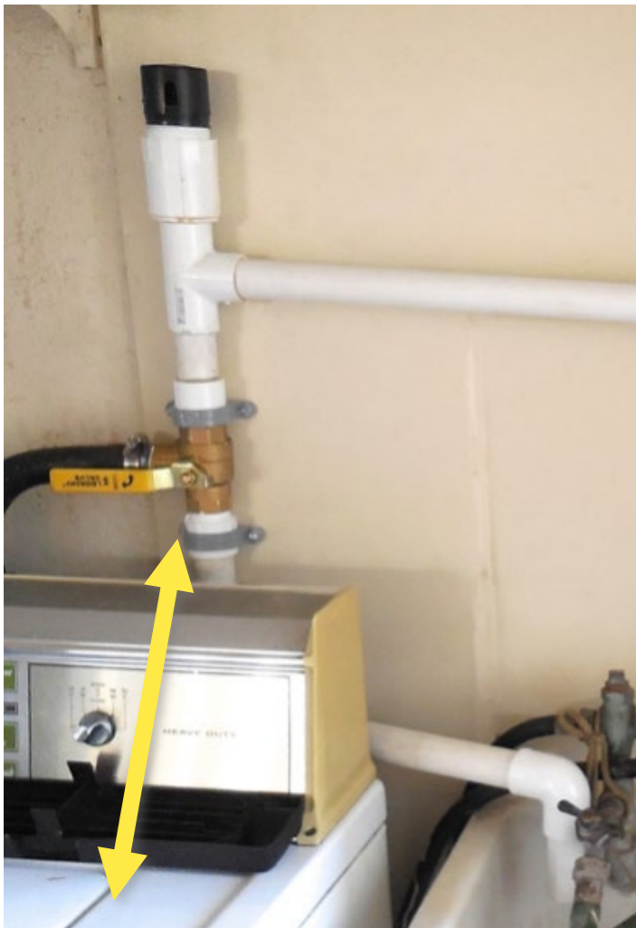
Washer hose connected to middle port
