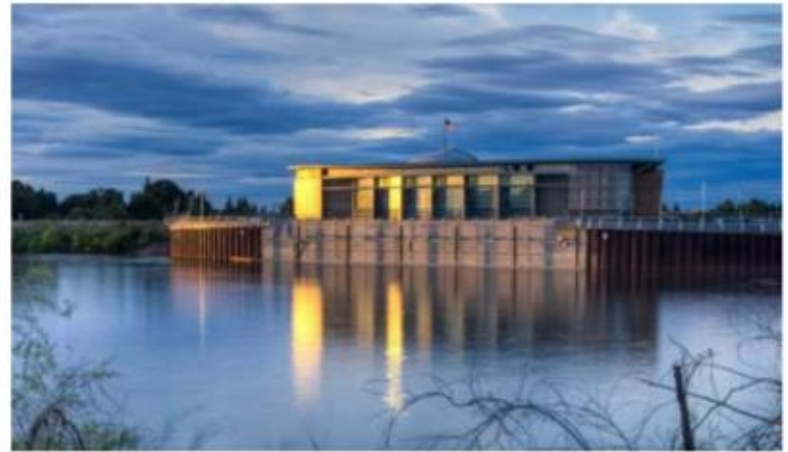
Freeport Intake Facility
