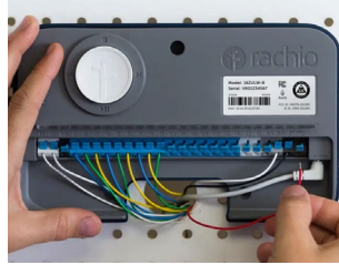
3) Installed new controller showing connected valve wiring
