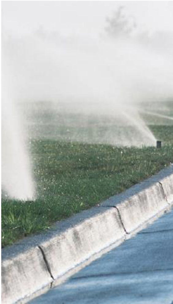
Before- Irrigation zone watered with inefficient fixed spray sprinklers that are causing misting, overspray and runoff.
