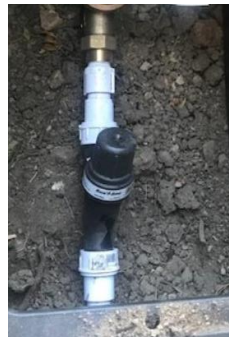
Drip pressure regulator and filter components
