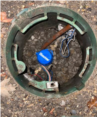
Photos of installed irrigation submeter, measuring only irrigation water. Include close-up to show leak detection feature (or screenshot of app if applicable).
