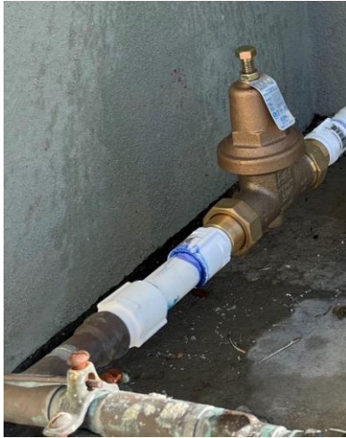
Photo of installed pressure regulator. Must be brass or bronze and installed upstream of entire irrigation system.
