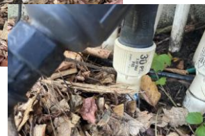
Drip pressure regulator and filter components
