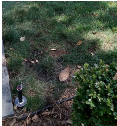
After- Irrigation zone watered with high-efficiency rotating nozzles.
