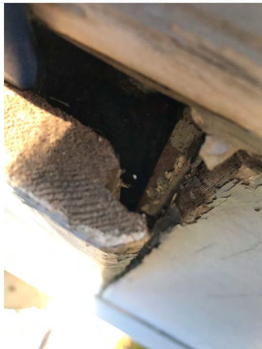
Tongue and Groove Siding
